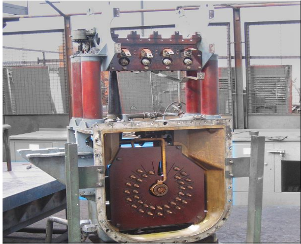
(A typical tap changer inside the transformer )
