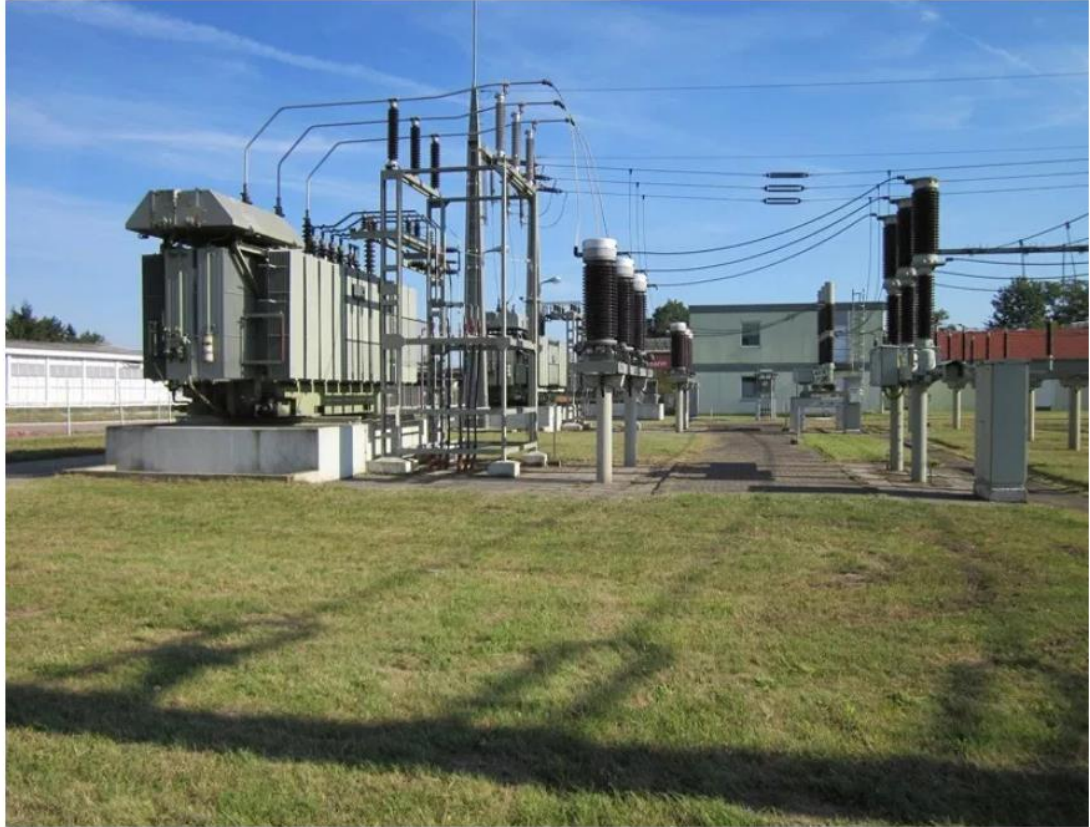
(parallel operation of Transformer)
